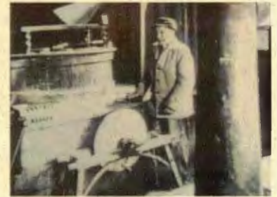
George Mayer on the Mill Platform
